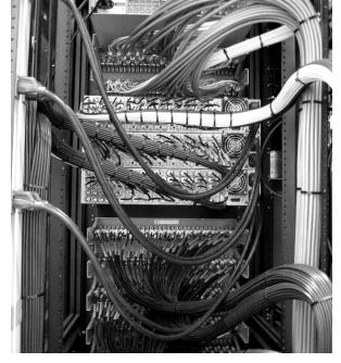
allow for service and testing. Provide horizontal support bars if cable bundles sag. Neatly bundle excess AC power cable from rack mounted equipment with velcro cable ties; where short power cables are not available. Rack wiring to be bundled with velcro cable ties. Electrical tape and adhesive backed cable tie anchors are not acceptable.
